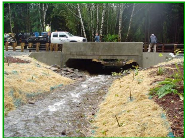
The newly installed three-sided box culvert increased the fish passage area from a 48" culvert to a 22' wide culvert, opening nearly two miles of upstream habitat.
