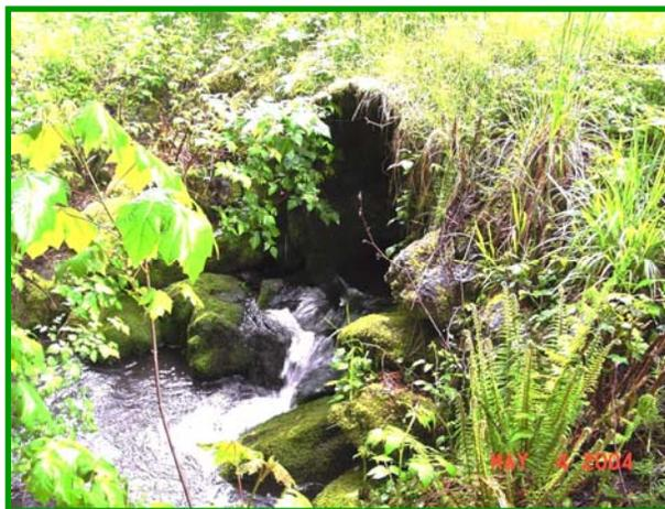
Dismal Creek culvert before replacement. This 4' diameter culvert created a fish passage barrier under the Upper Hoh Road.
